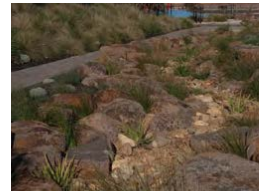
Rock stabilised embankment, revegetated where possible
