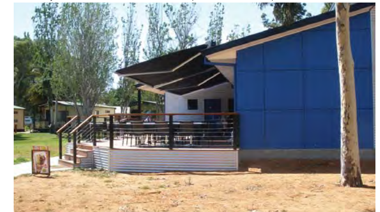
Recently constructed Caravan Reception, cafe and public toilets
