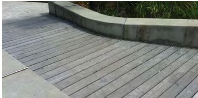
G.3 Timber decking / boardwalk
