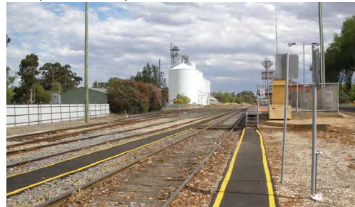
Railway corridor and adjacent rail uses
