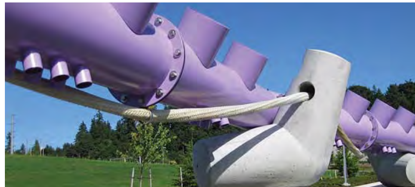
Demonstrating water / stormwater process
