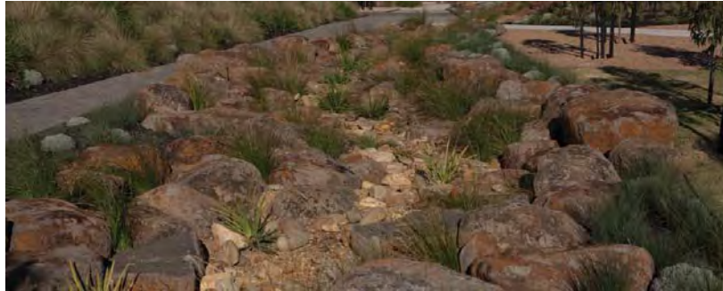
F.4 Dry creek bed that may temporary become inundated during peak flows
