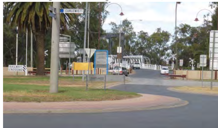
View of lift bridge from CBD (along McCallum Street)
