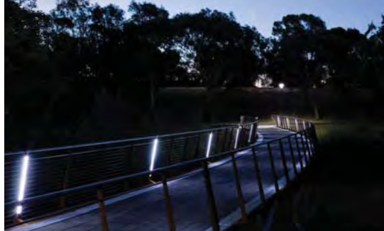
E.2 Lighting along bridge / boardwalk features
