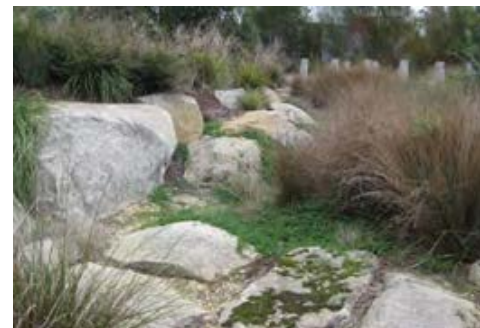
D.3 Rock stabilised embankment, revegetated where possible
