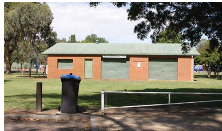
Canoe Club / Public Toilets in Riverside Park
