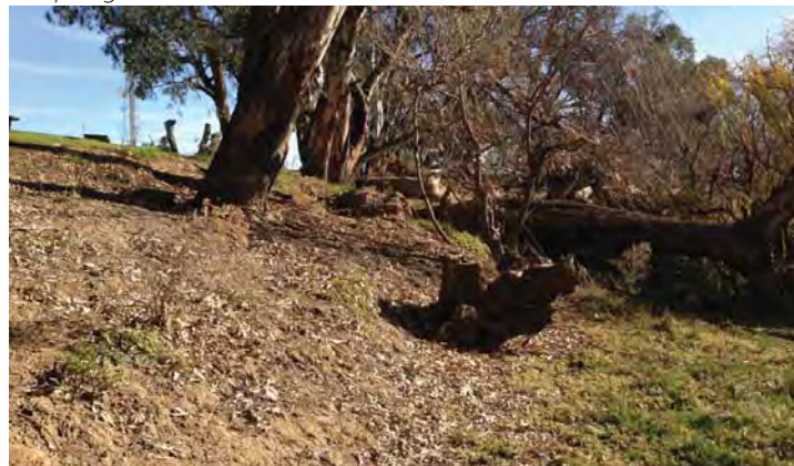
Steep degraded riverbank
