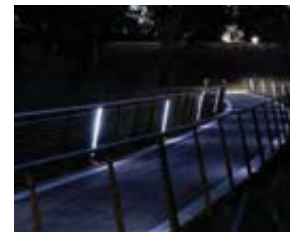
Footbridge / Boardwalk Enable people to safely cross the boardwalk / footbridge at night
