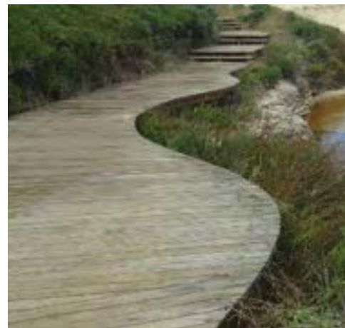
Timber boardwalk following form of embankment
