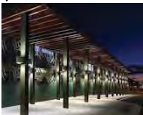
Transport Hub Lighting provides a good first impression of Swan Hill for people coming by train and improves passive surveillance
