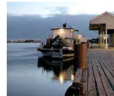
D.4 Wharf / Jetty
