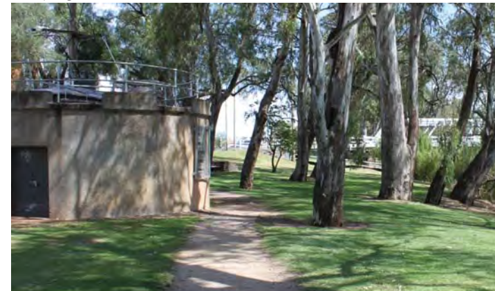
Pumping Station No.1 in Riverside Park
