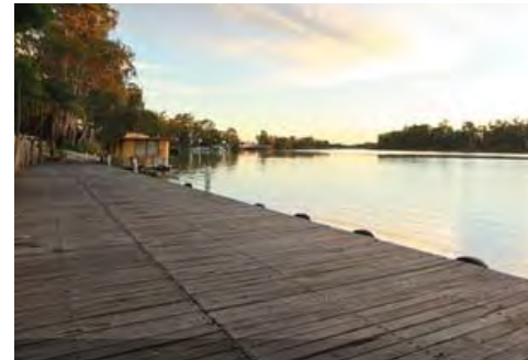
C.3 Timber boardwalk following form of embankment
