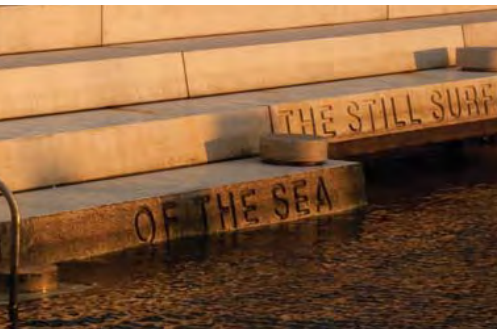
K.11 Steps to demonstrate water level changes and to reveal a message
