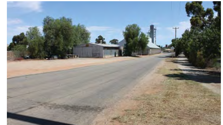
Monash Drive and views to Grain Corp silos / shed
