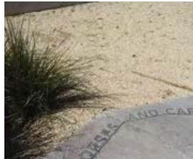
G.6 Gravel and uncoloured concrete
