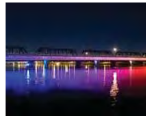
Swan Hill Bridge Lighting along bridge to emphasize this key feature at night
