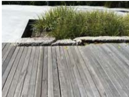
G.1 Timbers and recycled concrete
