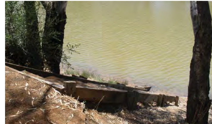
Rivers edge with timber steps to water
