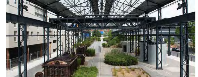
A.5 Existing structure, opened up for reuse as a public space
