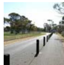
Bollards separating car traffic and pedestrian traffic
