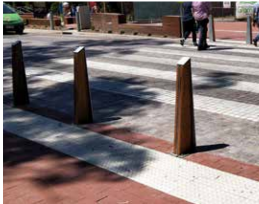
Raised crossing to provide a flushed kerb
