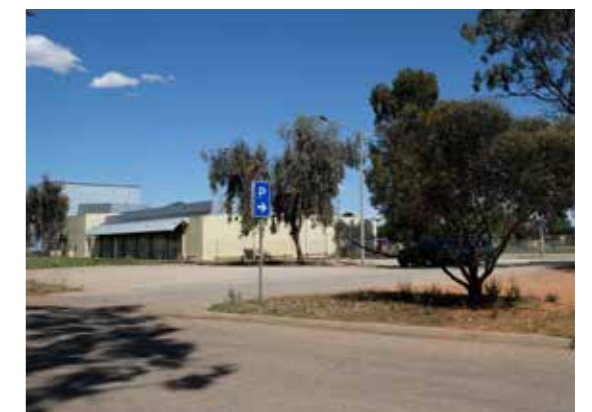
Existing carpark access
