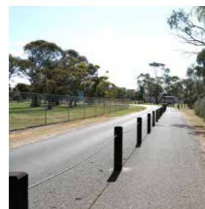
Bollards separating car traffic and pedestrian traffic
