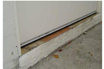
Pest strip fitted on external door
