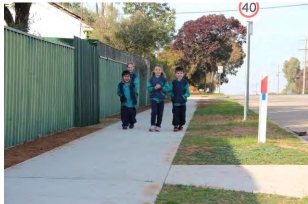
Recently constructed footpath in Nyah West
