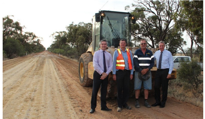
CEO Dean Miller, Civil Works Supervisor Ben Hawthorn, Coburns Earthmoving's Kent Coburn and Member for Swan Hill Peter Walsh at the Lake Boga-Ultima Road in March when the road was being widened with funding from the State Government's Country Roads and Bridges program.
