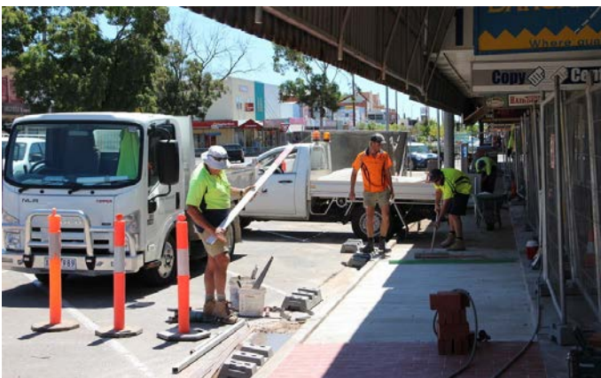
Council's works team and contractors during CBD Stage 3 work.
