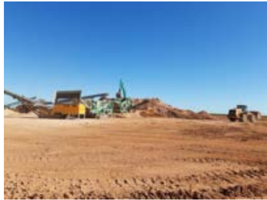
Figure 2 Example of crushing and screening equipment
