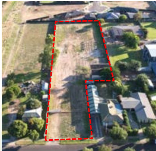
Figure 1 Subject site from Rutherford Street
