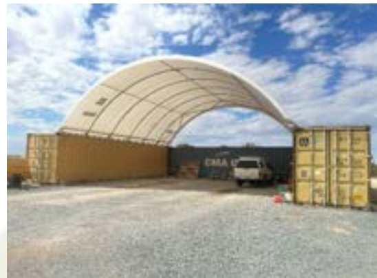
Figure 8 Temporary shade structure
