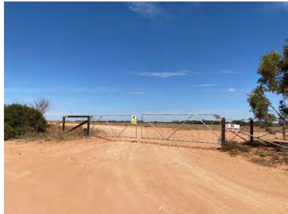
Figure 14 Existing double gate access
