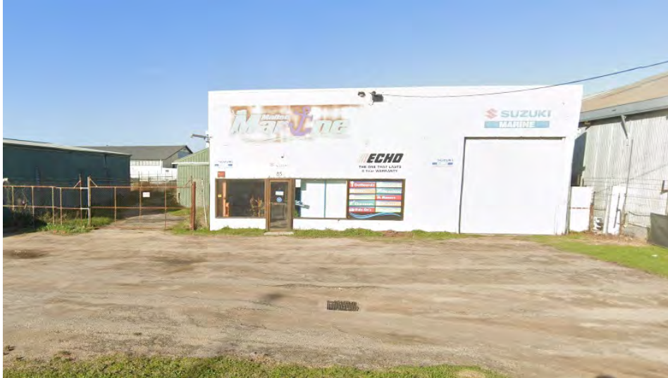
Picture 2 Existing frontage as at June 2023
