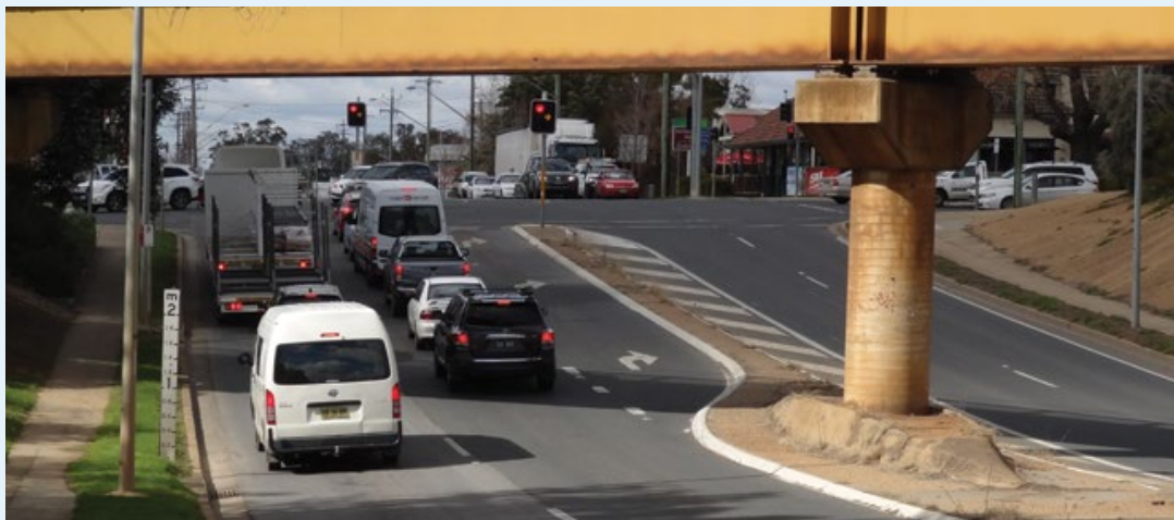
Figure 9. Traffic signals along the Sturt Highway at Lake Albert Road have been reprogrammed to improve traffic efficiency
