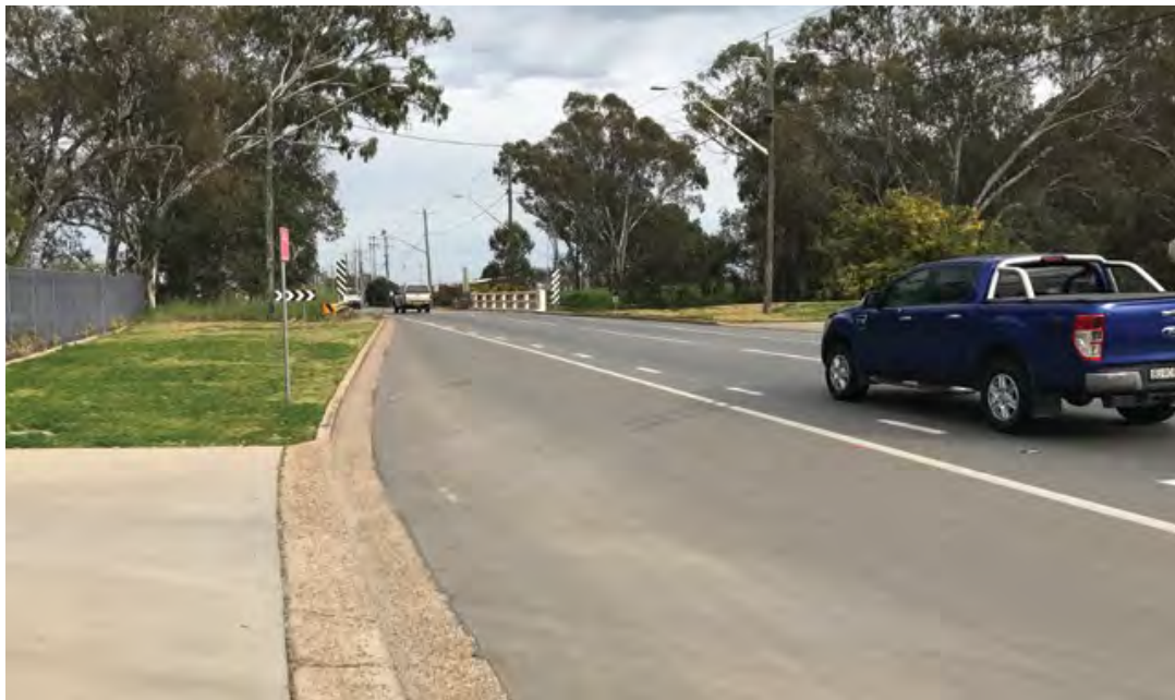
Figure 8. Planning work has started on widening the Sturt Highway at Marshalls Creek Bridge
