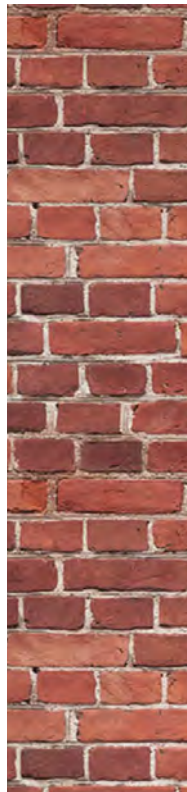
1. Pressed Reds Brickwork
