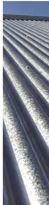
4. Heritage Zinc Roof Sheeting
