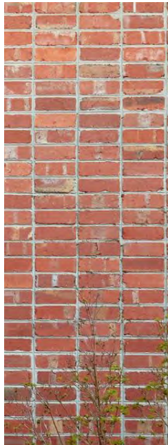
1. Red brick paver stacker bond
