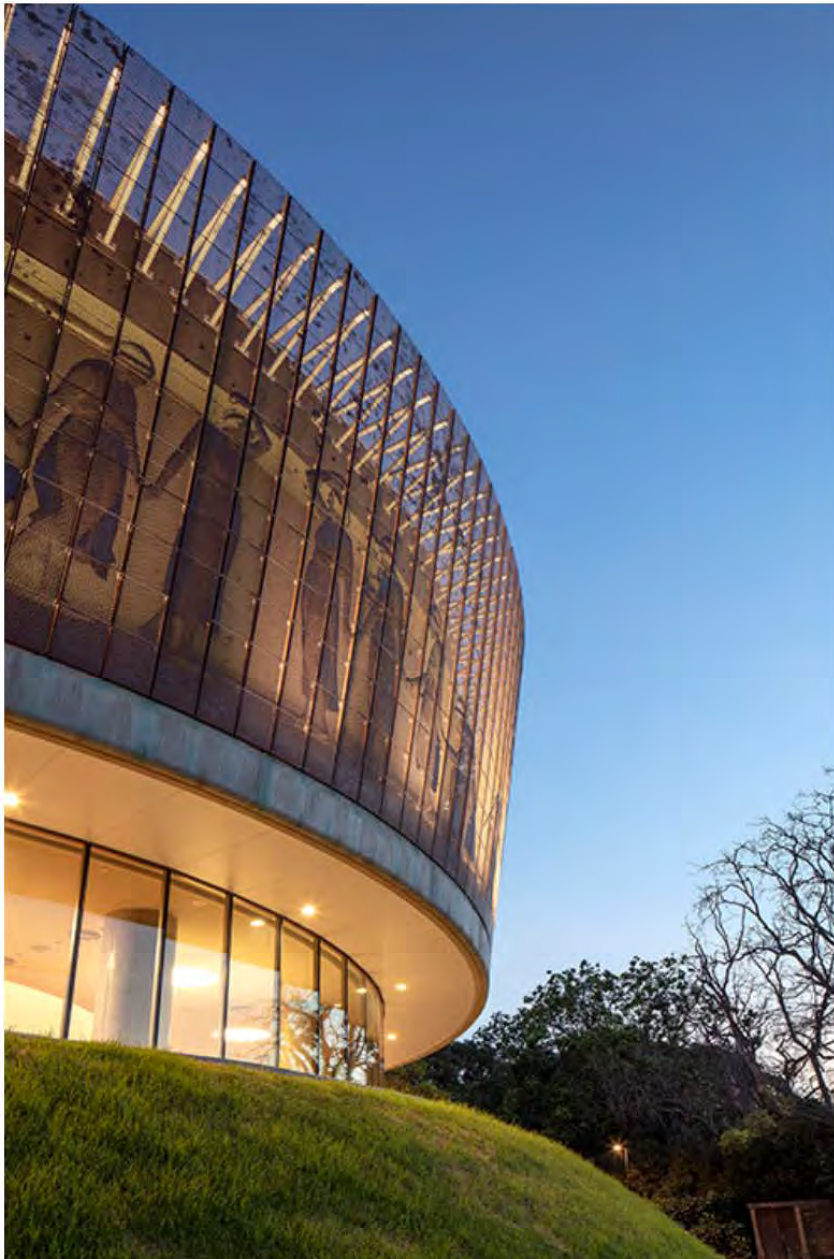
m3architecture, Facade depicting Greek figure Sybil. Perforated panel by Tensile. https://www.tensile.com.au/project/the-womens-college-copper-panel-facade/
