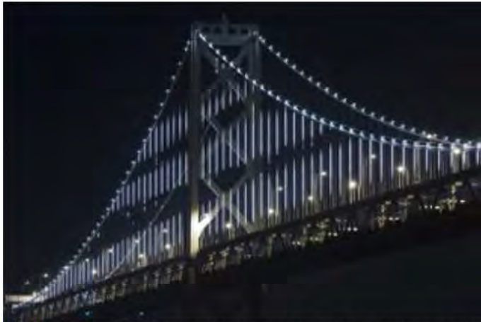
Leo Villareal , 2013. San Francisco Bay Bridge, “using equipment developed by Philips Lighting. The artwork, which originally appeared in March 2013 as a two-year installation, will now permanently illuminate the San Francisco Bay’s night sky 25,000 Philips connected light points and an advanced cloud-based connected lighting platform to remotely monitor and maintain the lighting system.” http://applications.nam.lighting.philips.com/blog/index.php/2016/01/28/artist-leo-villareal-shines-a-permanent-light-on-san-francisco-with-led-lighting-from-philips/
