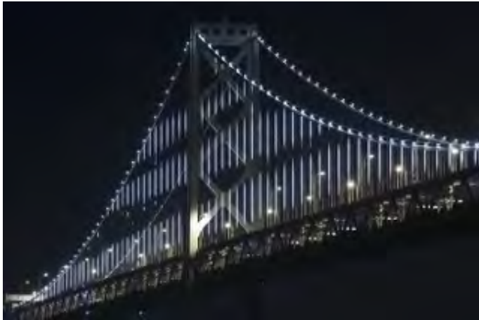
Leo Villareal, 2013. San Francisco Bay Bridge, “using equipment developed by Philips Lighting. The artwork, which originally appeared in March 2013 as a two-year installation, will now permanently illuminate the San Francisco Bay’s night sky 25,000 Philips connected light points and an advanced cloud-based connected lighting platform to remotely monitor and maintain the lighting system.”
