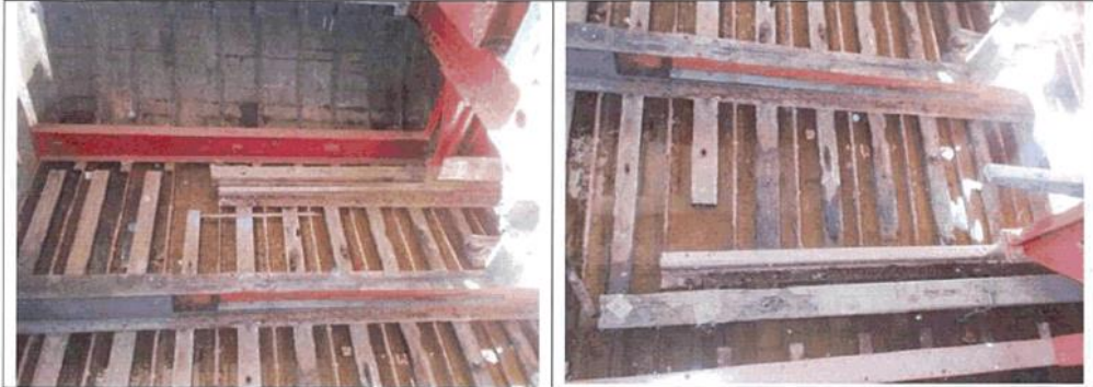
Keelson, sister keelsons, ribs, bilge stringers, in engine compartment
