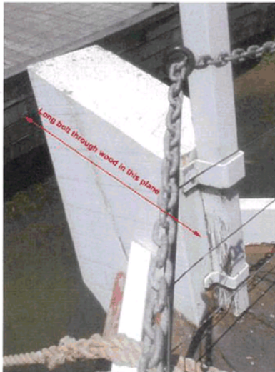
Repairs to Stem Post to reduce cracking
