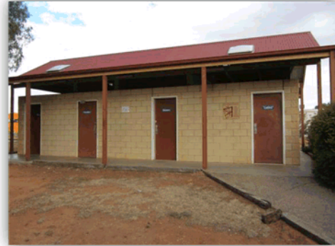
Photo 1 - Example of the use of Skylights
