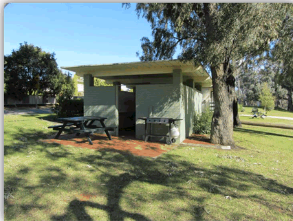
Photo 2 - Example of inappropriate positioning of street furniture
