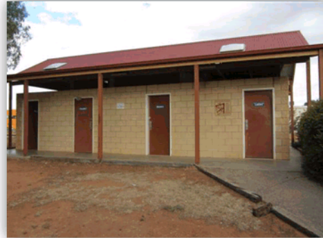
Photo 1 - Example of the use of Skylights
