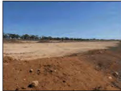
Plate 3: Existing pit, facing northwest (Photo: J. Bell 24Sept18)
