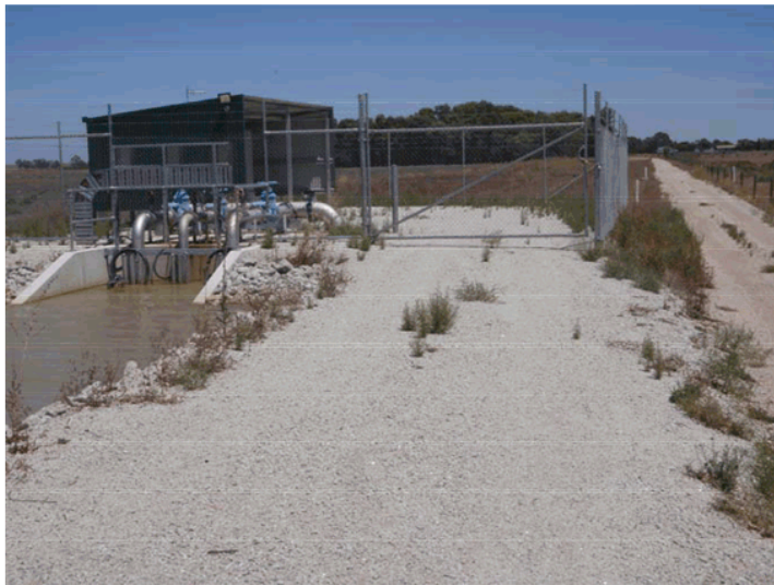
Photo 1 shows the compound near McKenzie Road.
