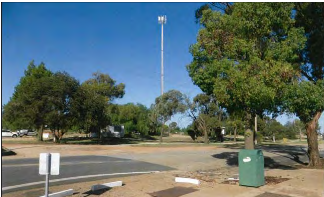
Figure 3. Photomontage – view of the proposed facility looking east from the corner of Marraboor Street and Station Street approximately 100 metres away.
