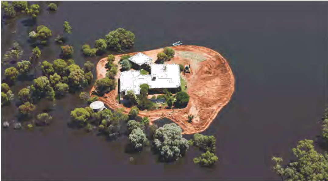
Ring levee at Culgoa, 2011.
