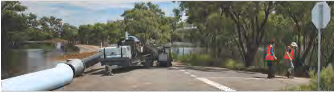
Pumping stormwater to restore access, Kulkynne Way 2011.
