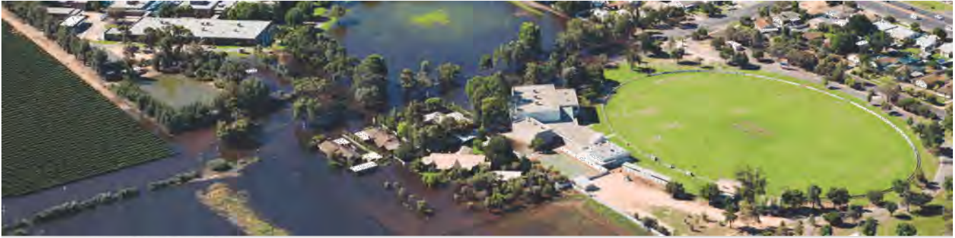
Stormwater Flooding, Irymple 2011.
