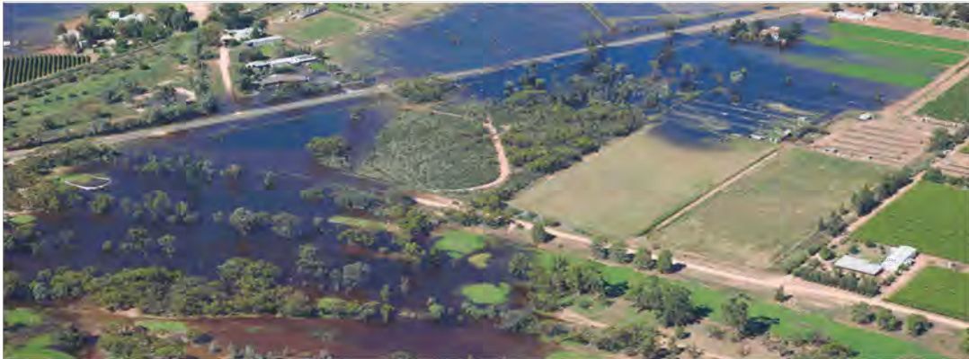
Stormwater flooding, Dow Avenue, Red Cliffs, 2011.
