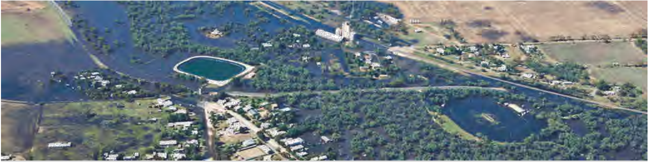
Tyrrell Creek flooding, Culgoa 2011.
