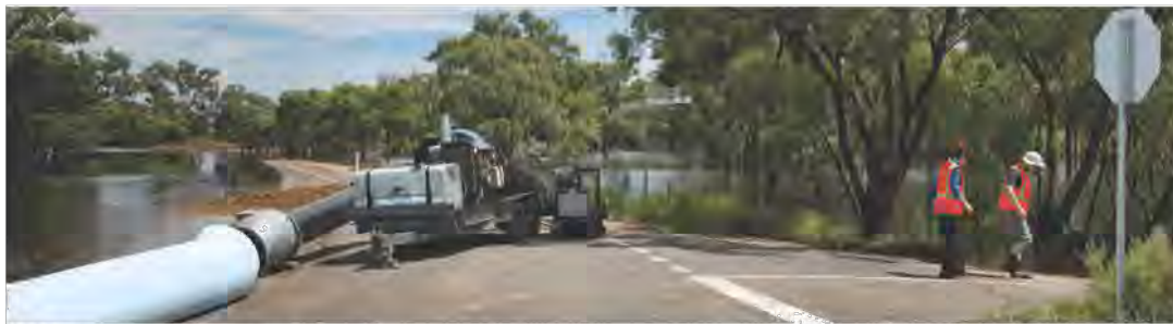
Pumping stormwater to restore access, Kulkynne Way 2011.
