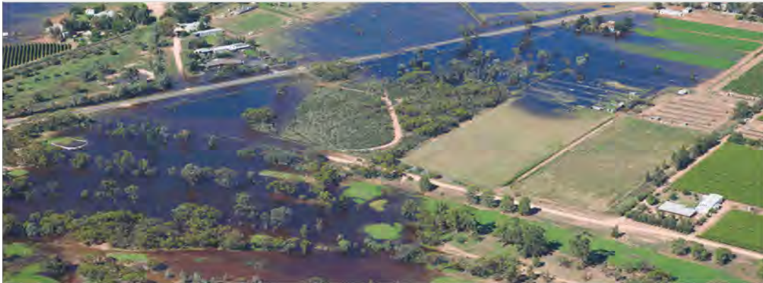
Stormwater flooding, Dow Avenue, Red Cliffs, 2011.
