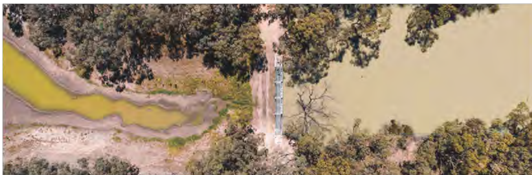
Beulah Weir on Yarrambiack Creek provides both flood mitigation and recreational benefits.
