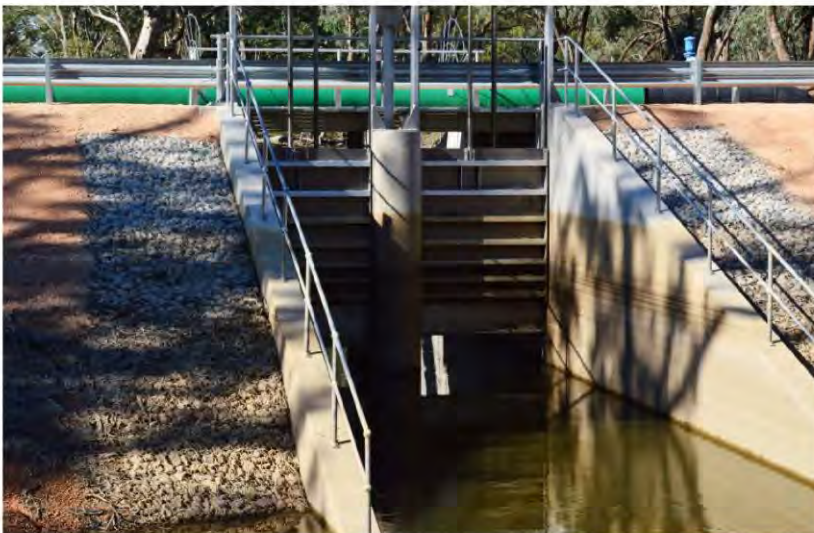
Above: Regulator with two gates in the down position at Messengers Bend
