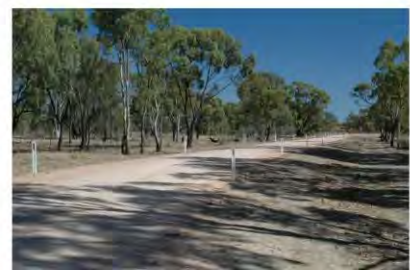
Above: Minor track raising at Hattah Lakes Photo: Mallee CMA.
