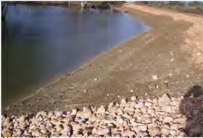
Above: Significant track raising at Mulca Island Photo: Mallee CMA.
